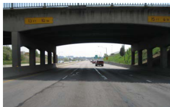
Existing Federal Boulevard Bridge over US 6
