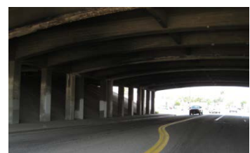
Bryant Street under US 6
