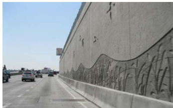
Alameda and I-25 wall treatments
