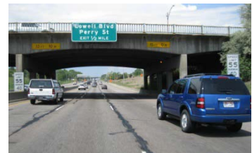
Westbound US 6 at the Federal Boulevard Bridge
